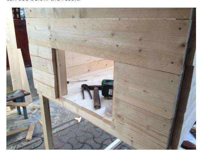
Using the boards  $10\frac{1}{2}$  in long, we will fix together those two wood boards  $16\frac{1}{2}$  in long in order to build the door. After this, using 2 hinges and a locker, we will fix the door up.
