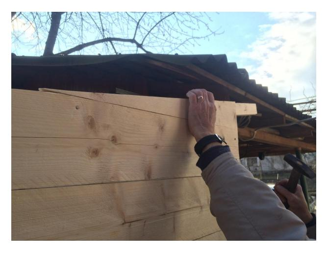
After doing this, we will now nail the boards in the bottom of the box. For this, we will need 4 boards 58 in long and 2 wood beams  $32\frac{5}{16}$  in long. We will nail two beams for a side of the box, and the other two for the other side, because right in the middle we will have the access door. Using the jigsaw cut the corners of the boards, so the board and the beam fit perfectly. I attached an image, this is how it should look.
