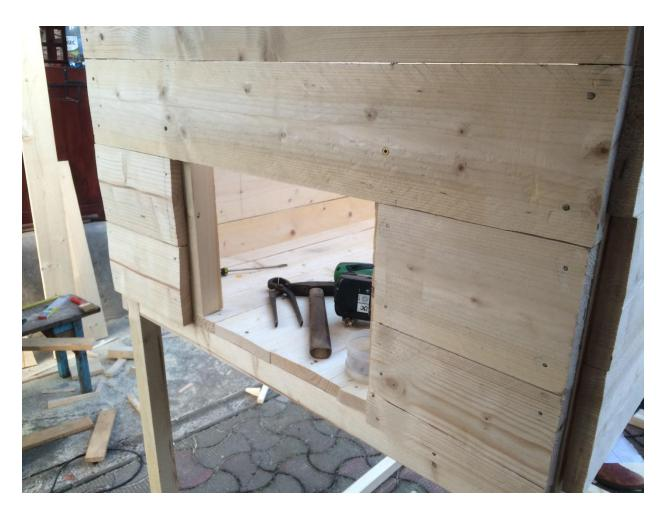
Using the boards 27 cm long, we will fix together those two wood boards 42 cm long in order to build the door. After this, using 2 hinges and a locker, we will fix the door up.
