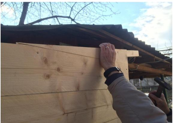
After doing this, we will now nail the boards in the bottom of the box. For this, we will need 4 boards 147 cm long and 2 wood beams 82 cm long. We will nail two beams for a side of the box, and the other two for the other side, because right in the middle we will have the access door. Using the jigsaw cut the corners of the boards, so the board and the beam fit perfectly. I attached an image, this is how it should look.
