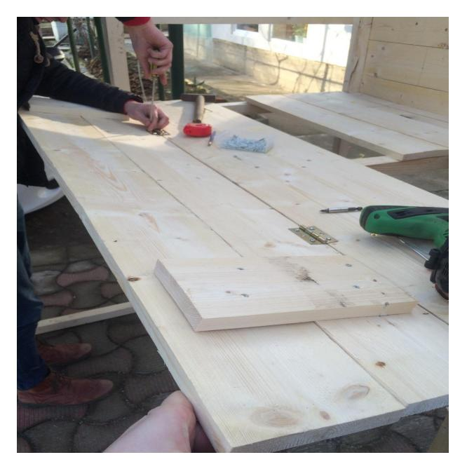
Then, we have to nail up the other boards over the door. We will need 4 more wood boards 59 in long. What remains now, is to fix the locker.
