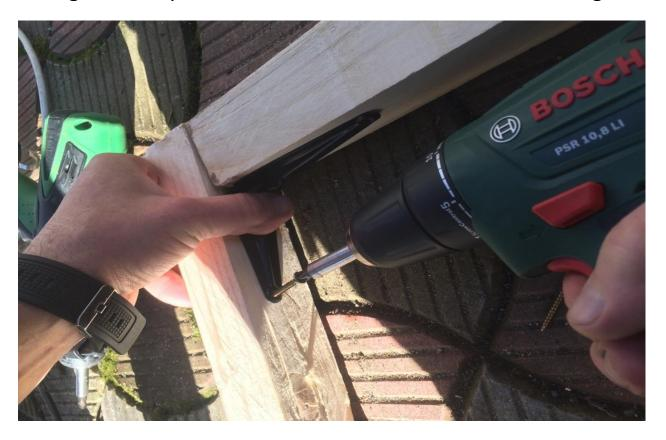
Now, we have to add two wood beams, parallel with bottom and upper beam. They have to be  $32\frac{5}{16}$  in long, and the one in the front should be placed at a distance of  $32\frac{5}{16}$  in under the top. The one in the back should be placed exactly over the one in the front, like in the image.
