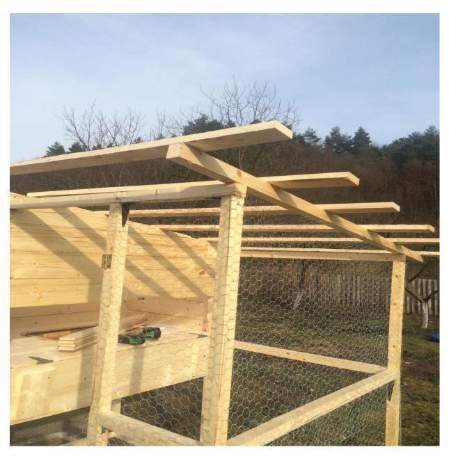
Now, using nails, the only thing remained to do is to fix the onduline over it.
