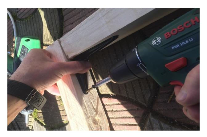
Now, we have to add two wood beams, parallel with bottom and upper beam. They have to be 82 cm long, and the one in the front should be placed at a distance of 82 cm under the top. The one in the back should be placed exactly over the one in the front, like in the image.
